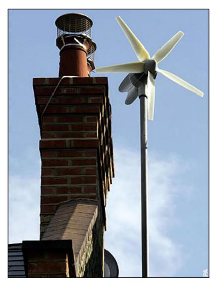
1.6 kWh/d if wind speed is 6 m/s
