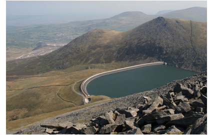
Figure 11. Marchlyn Mawr, the upper reservoir of the Dinorwig pumped storage facility. See Chapter 26 (pages 186–194) for further information.
