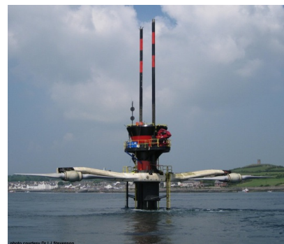
Figure 1.6. Seagen (Strangford Lough), the only grid-connected tidal stream device in the UK. Capacity: 1.2 MW. Photo by Dr. I.J. Stevenson.
