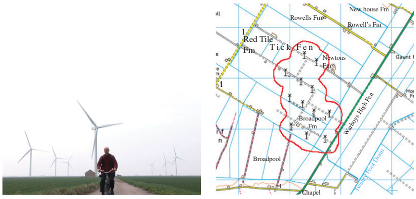
Figure 9. Red Tile wind farm, East Anglia and its associated land area. The blue grid's spacing is 1 km. Each turbine has a diameter of 82 m and a capacity of 2 MW. Map Crown copyright; Ordnance Survey. (Online version in colour.)
