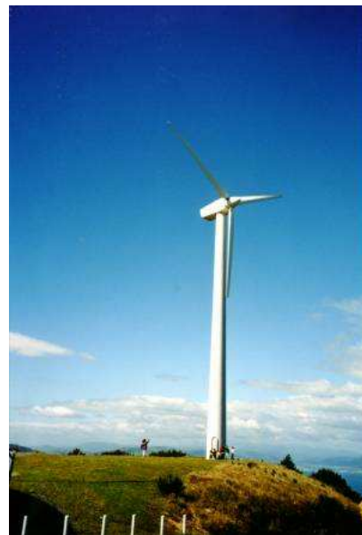
Figure 1.5. The Brooklyn windmill above Wellington, New Zealand, with people providing a scale at the base. On a breezy day, this windmill was producing 60 kW, or 1400 kWh per day. Photo by Philip Banks.
