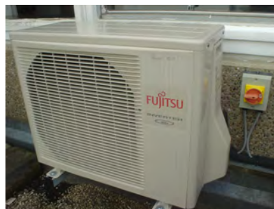
Figure 13. Good: The inner and outer bits of an air-source heat pump that has a coefficient of performance of 4. The inner bit is accompanied by a ball-point pen, for scale. One of these Fujitsu units can deliver 3.6 kW of heating when using just 0.845 kW of electricity. It can also run in reverse, delivering 2.6 kW of cooling when using 0.655 kW of electricity.
