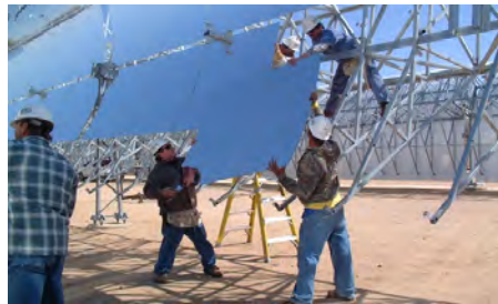
Figure 8. Andasol – a "100 MW" solar power station under construction in Spain. Excess thermal energy produced during the day will be stored in liquid salt tanks for up to seven hours, allowing a continuous and stable supply of electric power to the grid. The power per unit land area will be 10 \text{ W/m}^2 . Photo: IEA SolarPACES.
